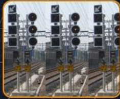
Signalling and Control
