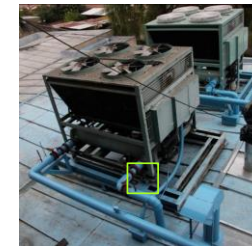
Anchored Equipment
