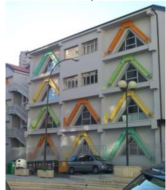
Seismic refurbishment of existing structures
