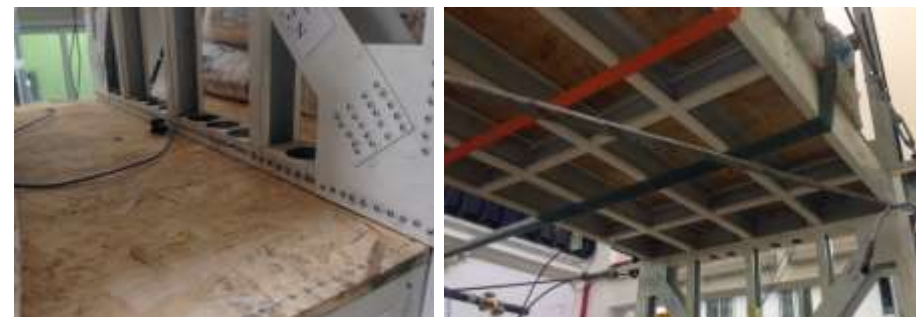
Prototype with wood-based (OSB panels) sheathing braced floors
