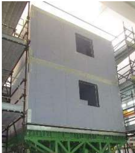
Whole bare structure
