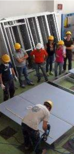
Exterior wall panels nailing
