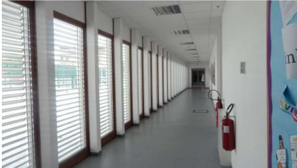
Interior partition wall
