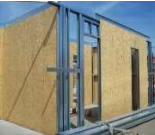
Sheathing- braced structure
