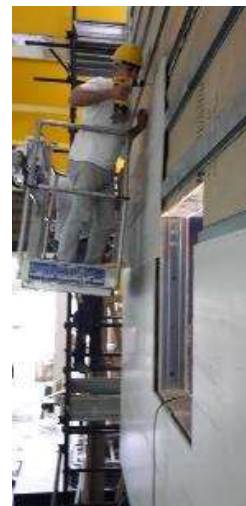
Exterior wall panels fixing
