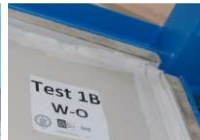
9. Rupture of panel portions
