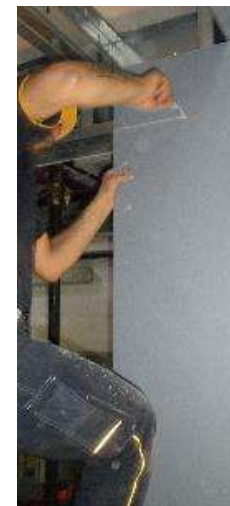
Interior wall panels fixing
