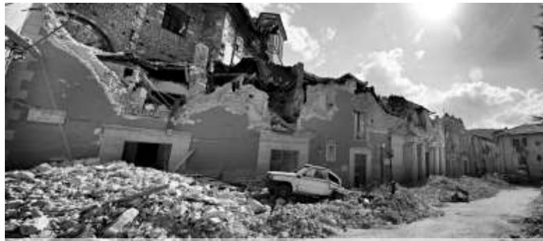
Damage caused by Aquila earthquake on traditional buildings
