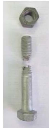
HR Bolt failure
