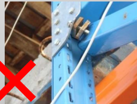
a. IPB – bracing connection failure
