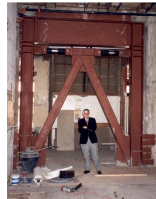
Seismic Dampers installed at the Hotel Woodland, in Woodland, California Force = 100,000 lbs., Stroke = +/- 2 inches Production = 16 pieces
