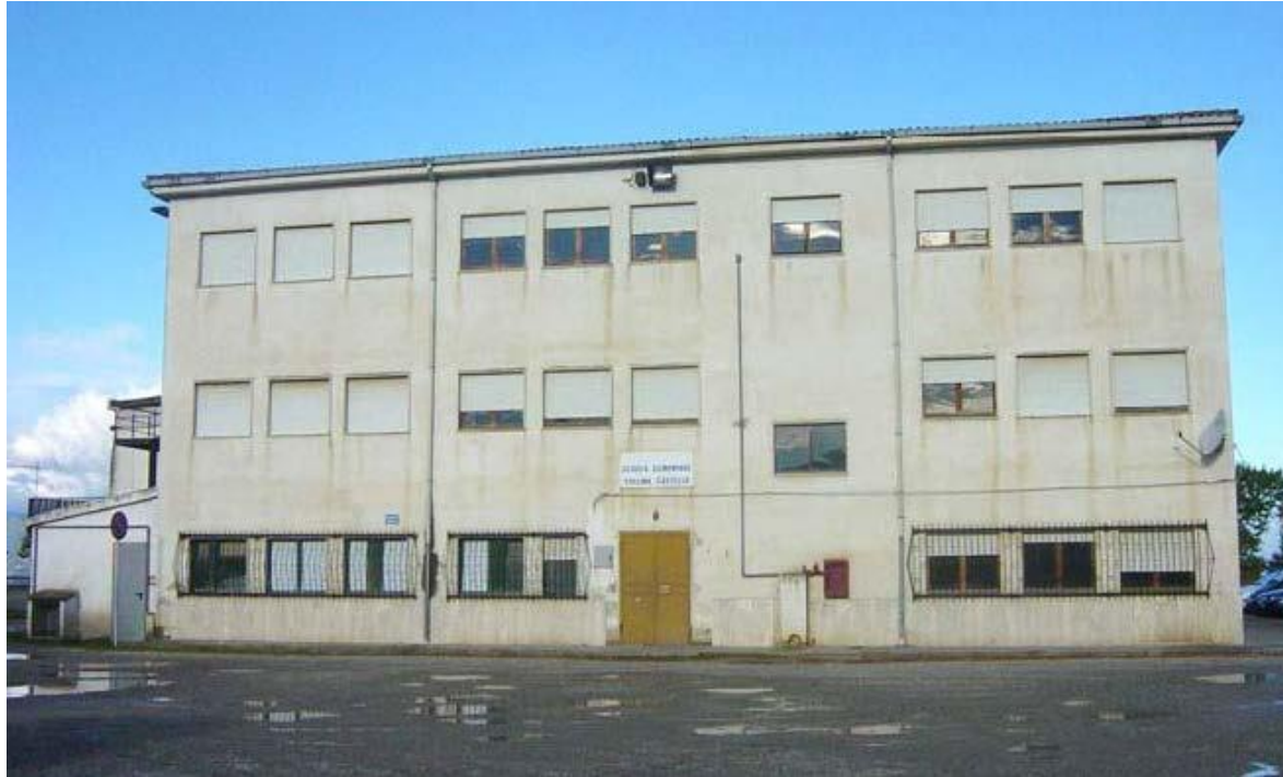
reinforced-concrete 3-storey school building located in Bisignano (Cosenza, southern Italy)
