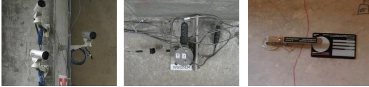
Measurement of deformations and crack widths
