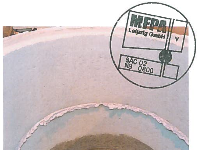
Pictures 3 and 4: View of the manhole rings after assembly with foam outlet on the outside and inside
