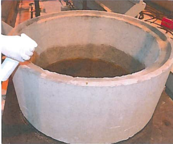
Pictures 1 and 2: Pretreatment: moistening the fold of a manhole ring SR-F DN 1000 x 500, Application of the polyurethane rigid foam on the fold
