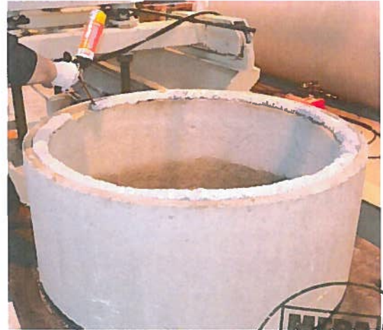
Pictures 1 and 2: Pretreatment: moistening the fold of a manhole ring SR-F DN 1000 x 500, Application of the polyurethane rigid foam on the fold
